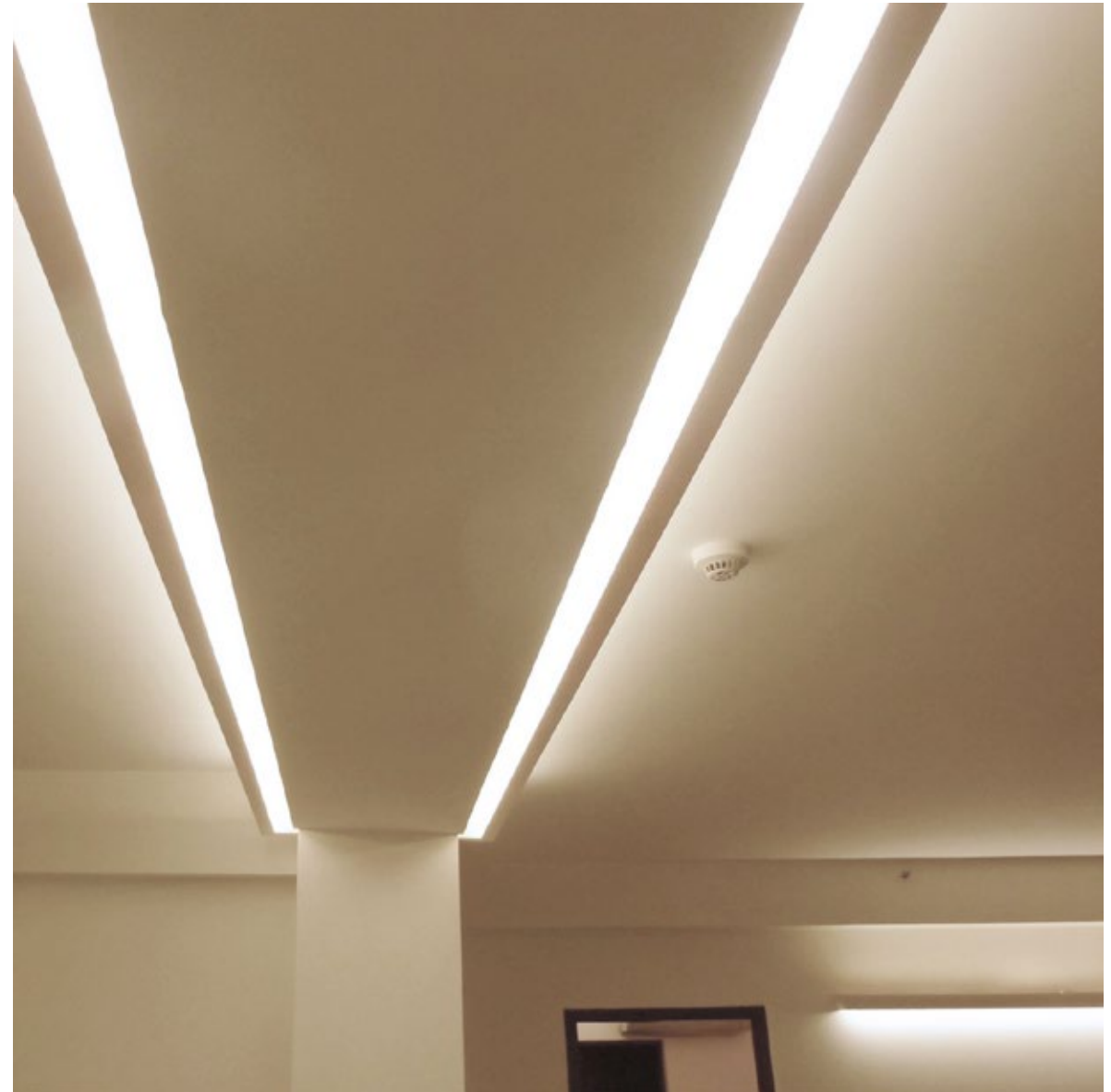
RL.cornice lighting profile mounted on both edges of a beam. Apartment, New Delhi
